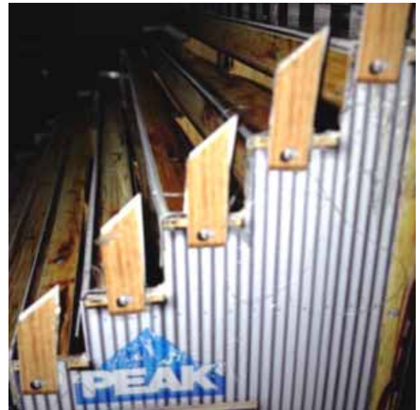
Figure 9 - Attach the handrail supports.
