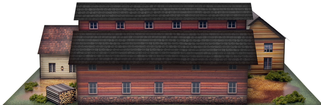
Rear of Buildings
